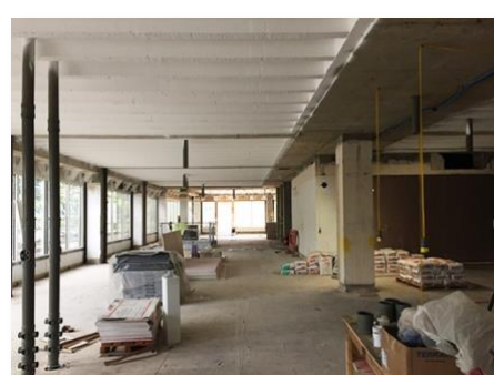
Westgate House: ribbed slabs protected with AITHON A90H
