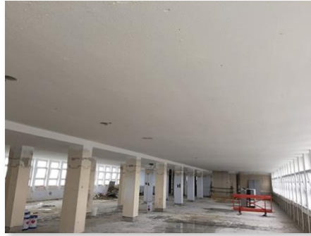
Europa House: slabs and columns protected with AITHON A90H
