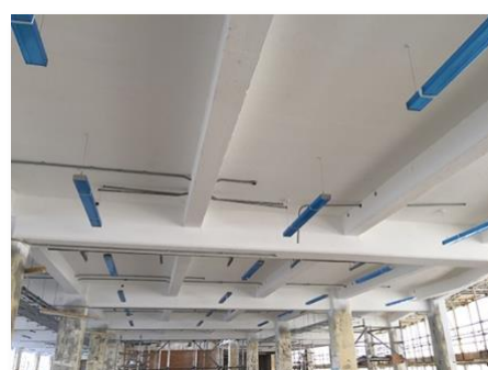
Old Vinyl Factory: beams and slabs protected with AITHON A90H
