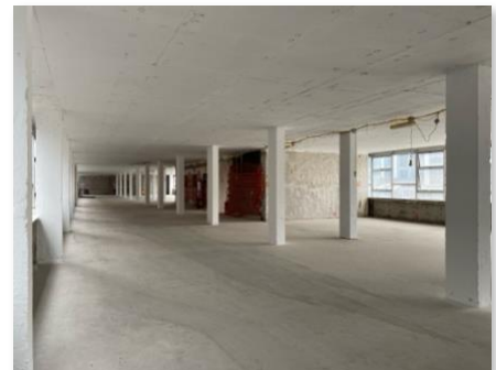
Old Granada Stuidios: slabs and columns protected with AITHON A90H
