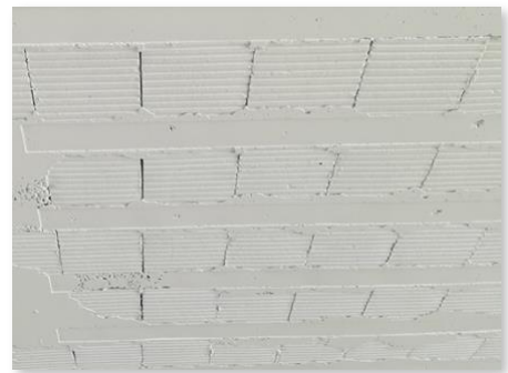
9 Millbank: potted slabs upgraded to R120 with AITHON A90H
