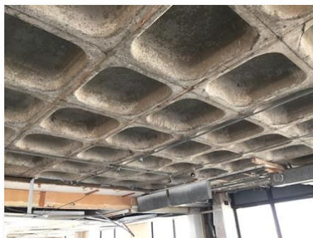
Echo Building: waffle slabs before the treatment
