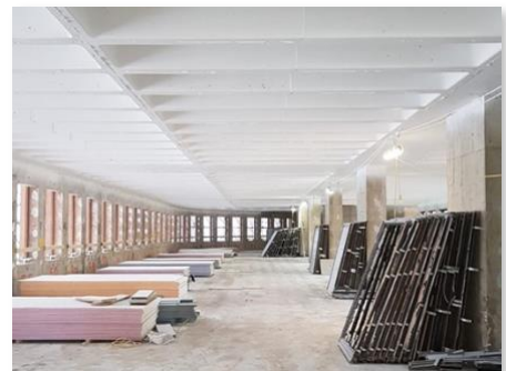
Hilton Canopy Hotel: Waffle slabs protected with AITHON A90H
