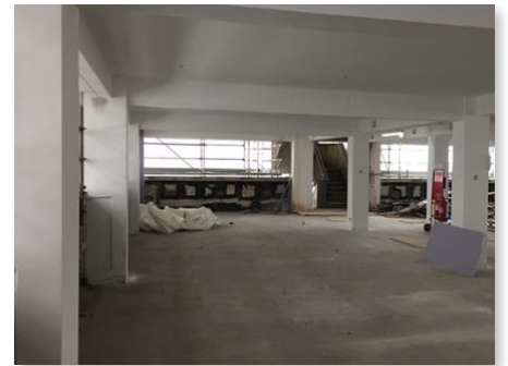
Bath Court: slabs, beams and columns protected with AITHON A90H
